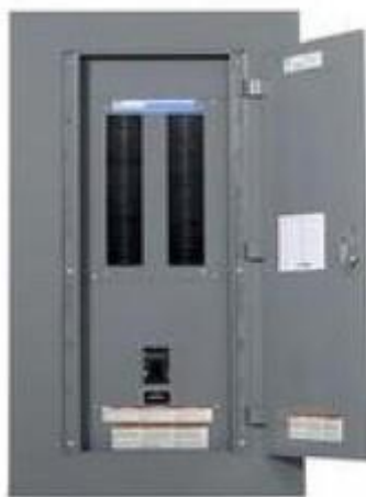
Figure 22 Photo of typical data center wall-mounted panelboard.
