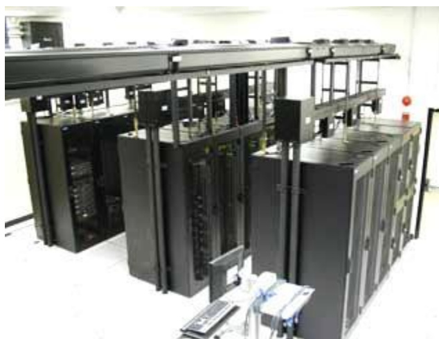
Figure 23 Example of a modular busway system.
